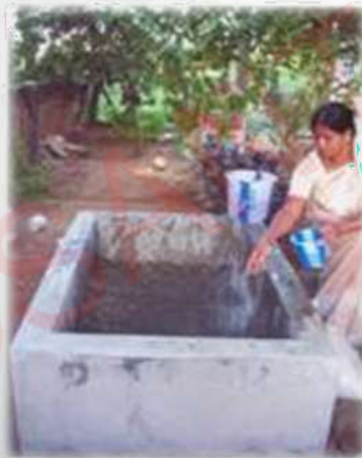
2. Sprinkling of water in tank with vermiculite
